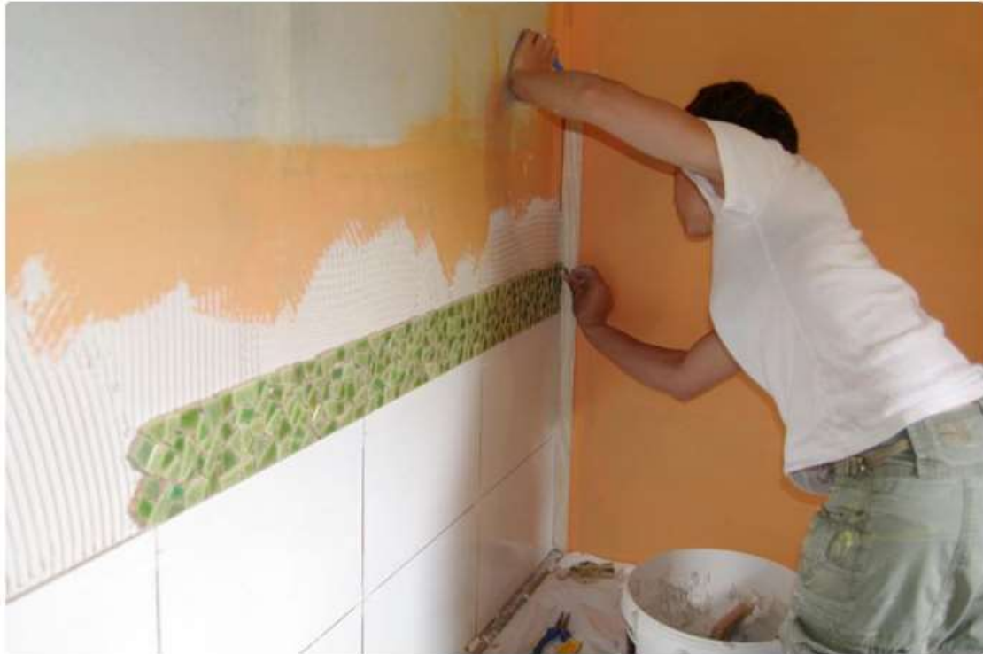
pose de carrelage - façade murale ©Fotolia
